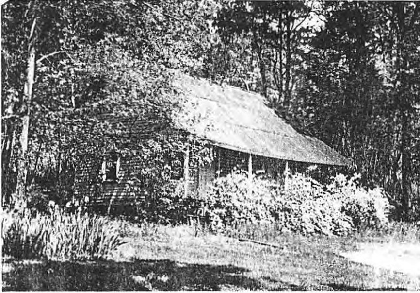
The two-room servants quarters cabin dates from the early days of the Christian plantation and possibly predates the house.
